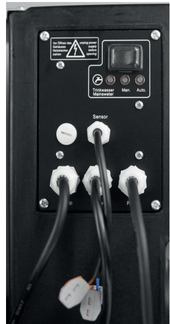
Fig. 8.8.1 Connection float switch
